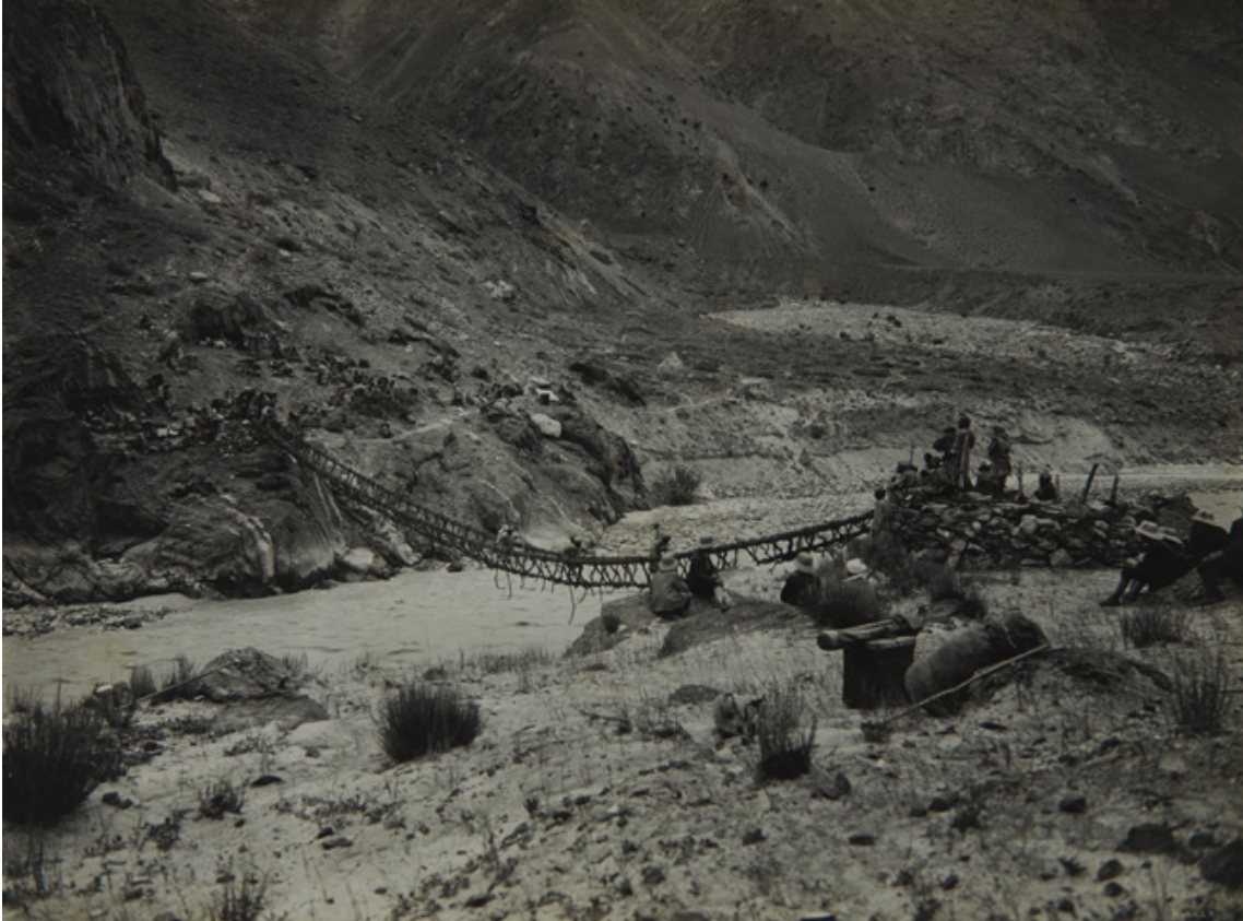
HK.266 – Rope Bridge on Punmah River
